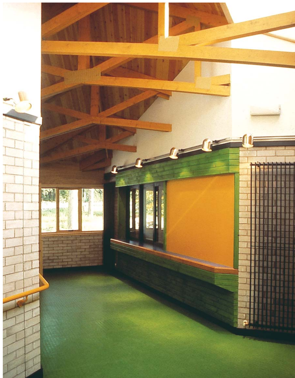
Roof trusses and ceiling cladding finished with Kiva Interior semi-matt Lacquer. Redwood lining boards to wall areas finished with tinted Kiva Interior semi-gloss Lacquer.
