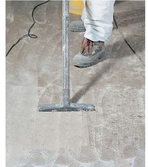
2. Removing dust with a vacuum-cleaner.
